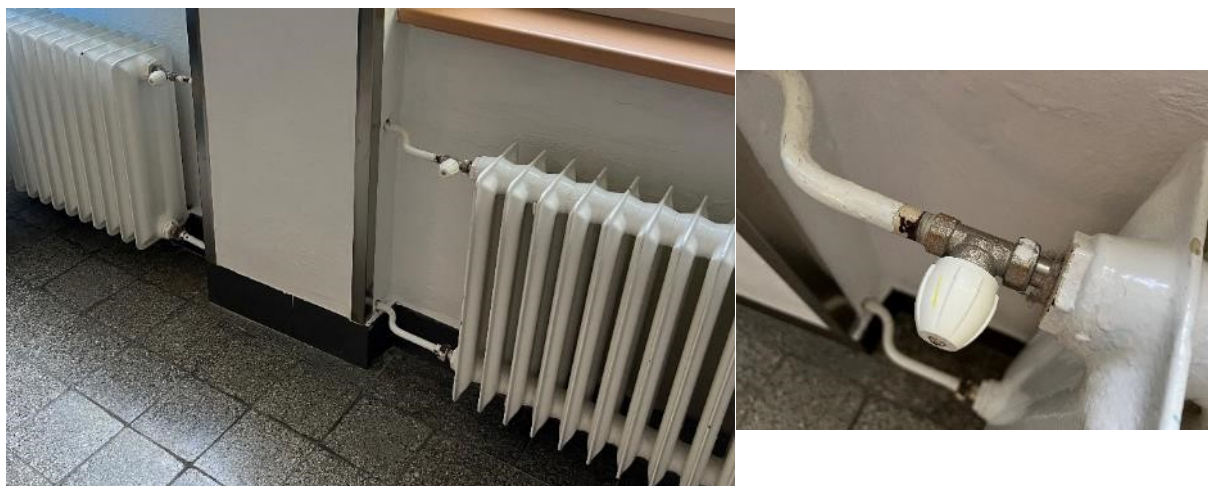
Obr. Detail OT a ventilu
