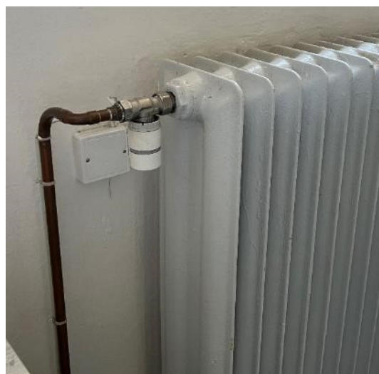
Obr. Detail OT v kabinetu – IRC hlavice
