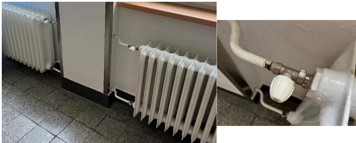
Obr. Detail OT a ventilu
