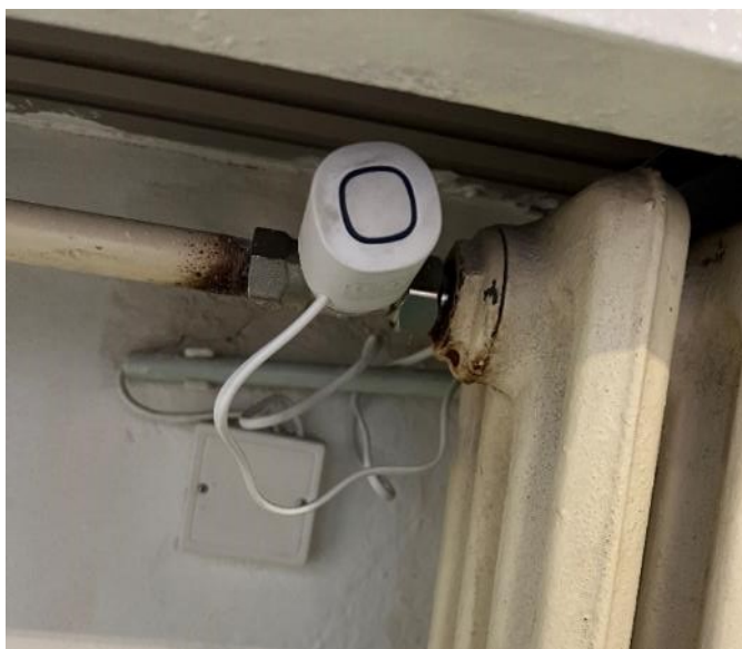
Obr. Detail IRC hlavice
